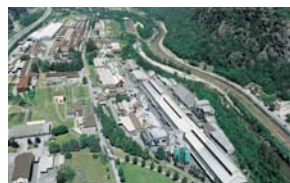
HQ Bodio, Switzerland Graphitization and processing of synthetic graphite, manufacturing of water-based dispersions, processing of natural graphite and coke, and manufacturing and processing of silicon carbide
